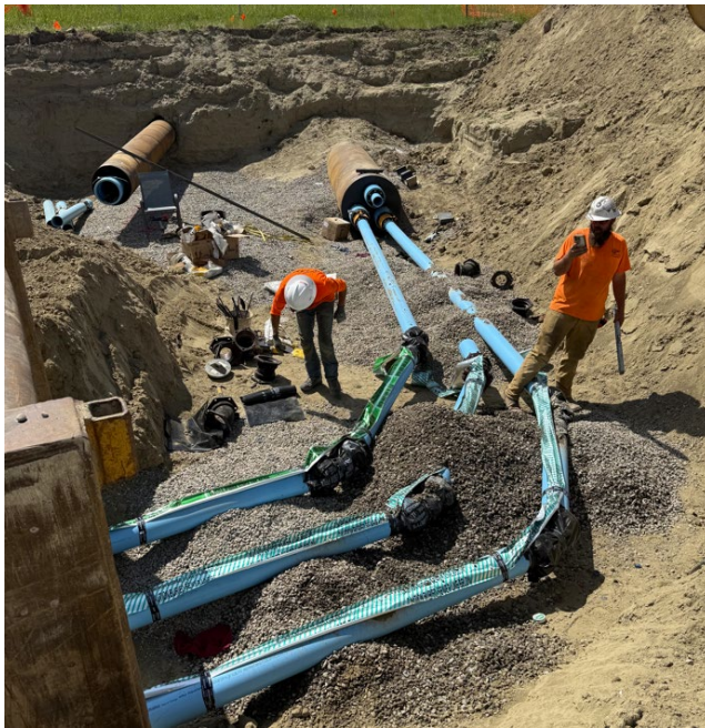
Left photo: 6/26/25, installation of the triple force main on the north end of the 42" interstate bore Right photo: 6/30/25, fire hydrant installation near the Town Pump
